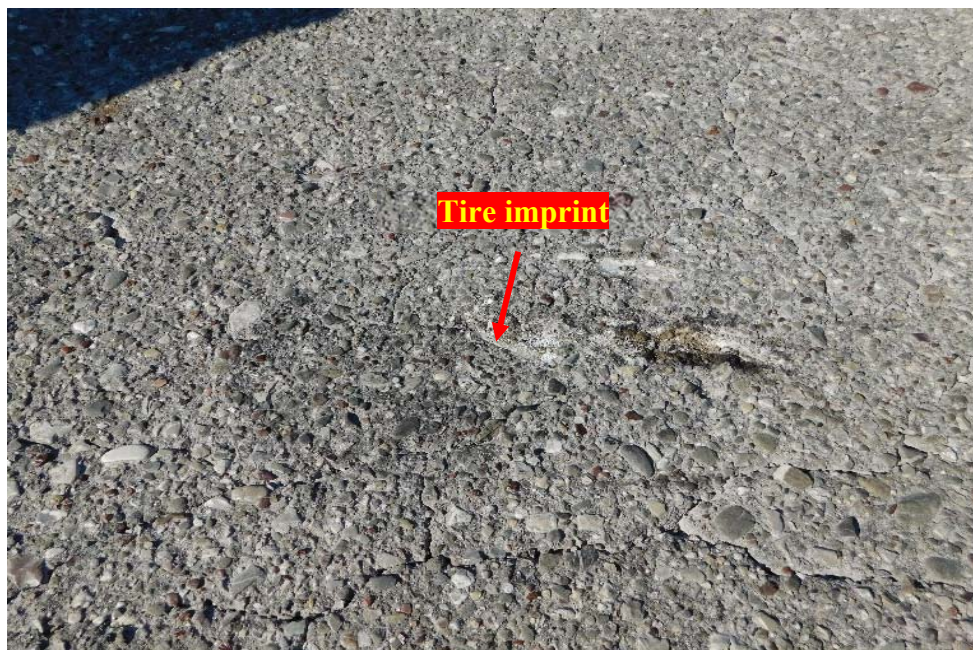
Photo 13: Imprint of the starboard tire on the road.
