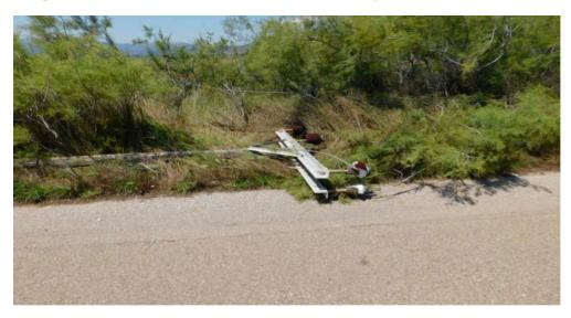
Photo 3: The power transmission pole, on the ground, following the impact
